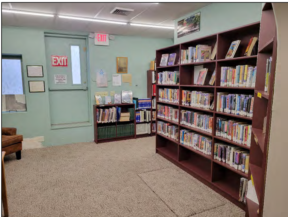
Photo 10. April 11, 2023. Street level. "Montana Room" with access to one section of the basement and emergency exit. Green plaster walls with ceiling tiles. Minor amount of loose insulation above ceiling tiles. Basement has drywall storage rooms, peg board, brick columns, and painted concrete.
