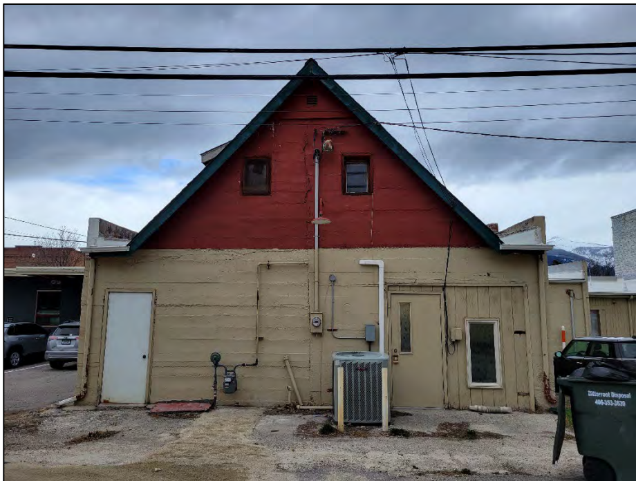
Photo 6. April 11, 2023. Outside looking west: ally side of the “Montana room” (tan room), boarded up storage closet (white door), and utilities (natural gas, electrical, telephone, and cooling) penetrating wood exterior walls. The southern and northern walls are concrete. Roofing (asphalt on pitch and membrane east to west sides) drainage discharging into gutters then onto the ground surface.
