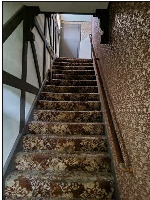
Photo 16. April 11, 2023. Stairwell to first floor above main library portion of the building. Carpeted stairs with wallpaper covering plaster walls on the right side and concrete walls on the left side. Doorway on top of stairwell leads to storage area.
