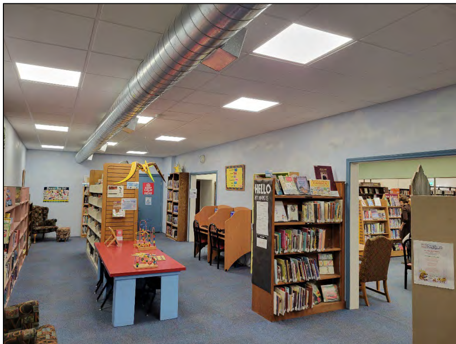
Photo 12. April 12, 2023. Street level. Kids room. Light blue painted drywall and ceiling tiles, same materials that are present in the computer station room. Concrete beneath carpet.
