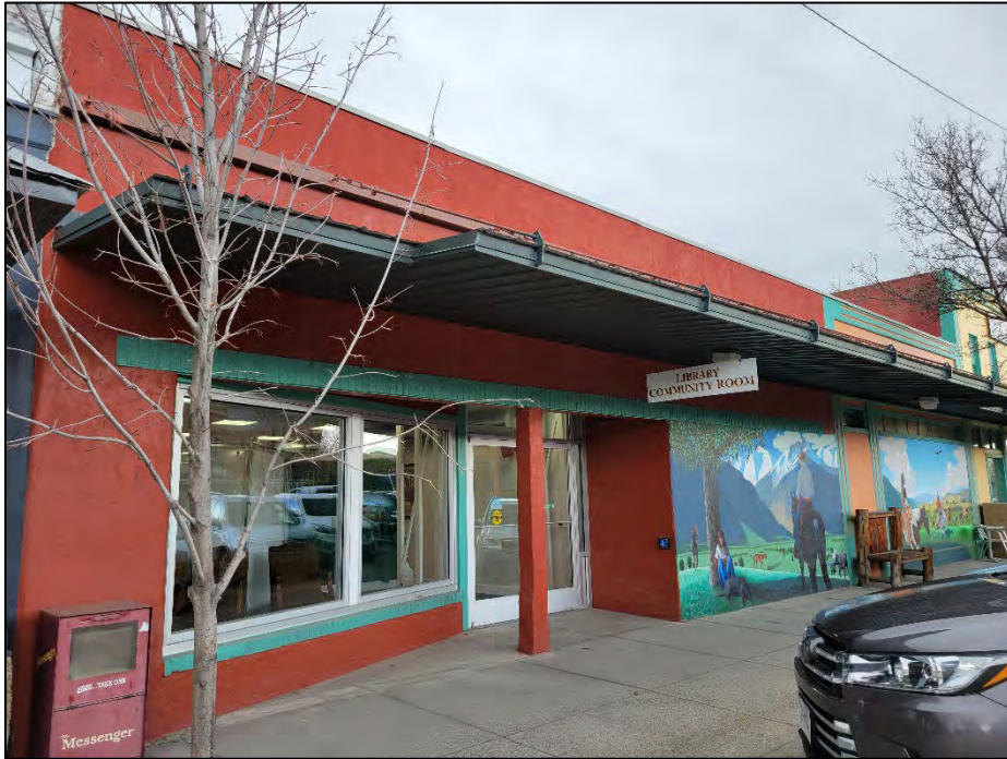
Photo 3. April 11, 2023. Outside looking southeast: Community room entrance.
