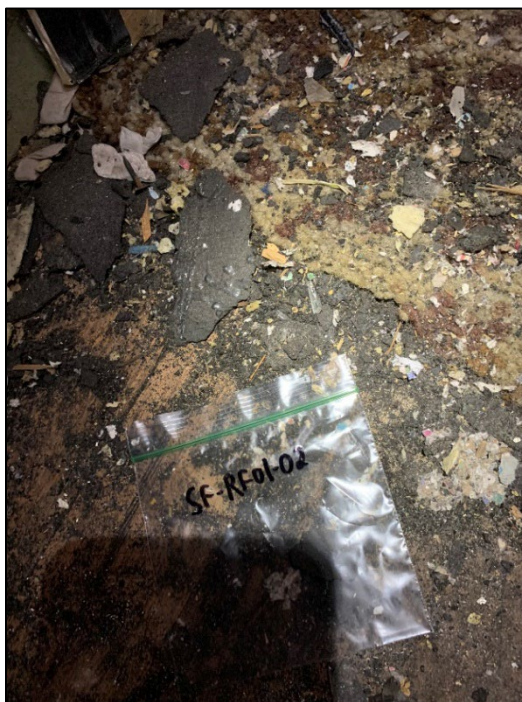
Photo 43. RF01: Asphalt roofing material in first floor storage room floor
