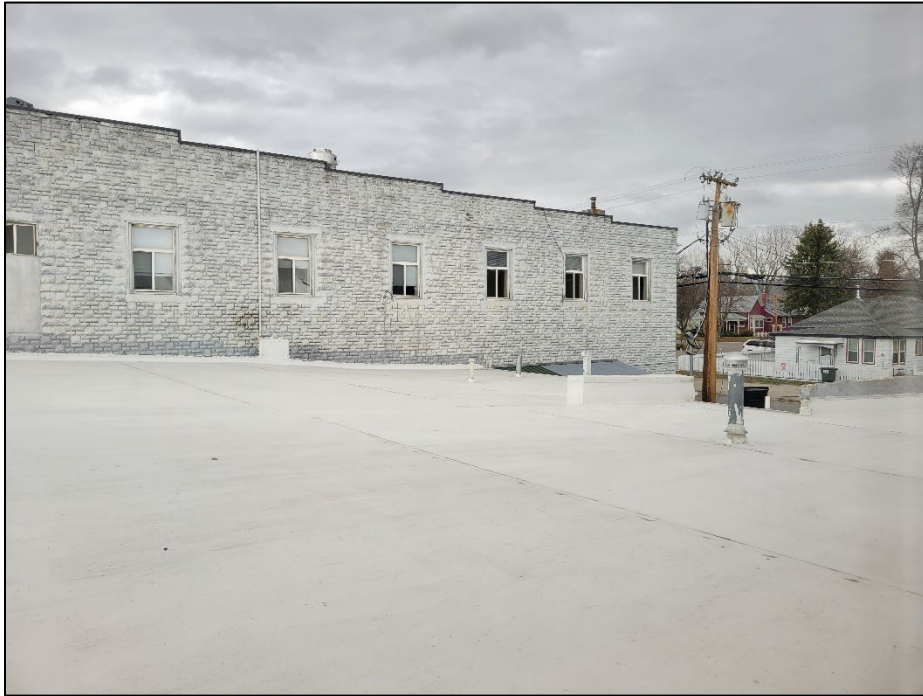
Photo 7. April 10, 2023. Outside on roof. Looking northeast from on the central building roof: Run off drains eastward towards the alley, is collected in gutters, before being discharged into the dirt park area.
