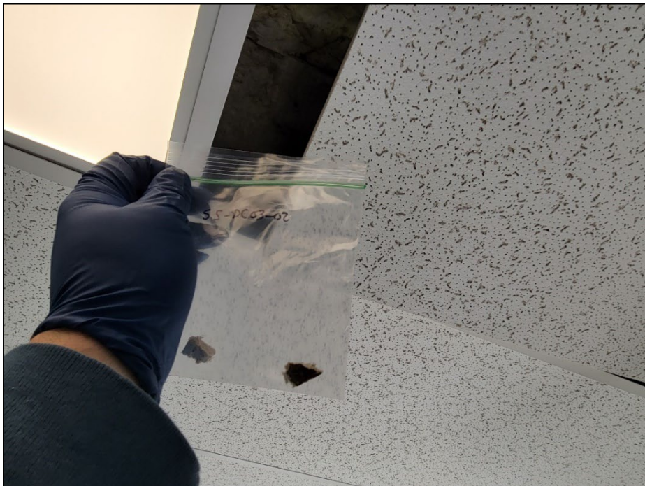
Photo 12. DC03: Drop ceiling in furnace / art room
