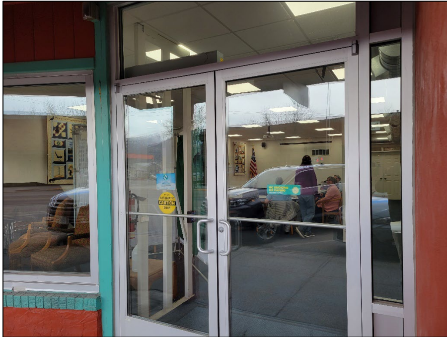
Photo 13. April 11, 2023. Street level. Community room with meeting taking place. White painted plaster / drywall and ceiling tiles. The drywall and ceiling tiles are the same materials as in the computer station and kid's rooms. Concrete beneath carpet.
