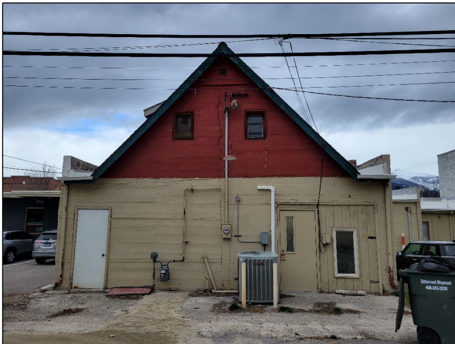
Photo 6. April 11, 2023. Outside looking west: ally side of the "Montana room" (tan room), boarded up storage closet (white door), and utilities (natural gas, electrical, telephone, and cooling) penetrating wood exterior walls. The southern and northern walls are concrete. Roofing (asphalt on pitch and membrane east to west sides) drainage discharging into gutters then onto the ground surface.
