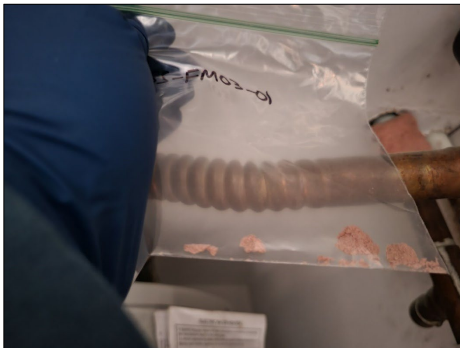
Photo 23. FM03: Pink spray foam next to water heater
