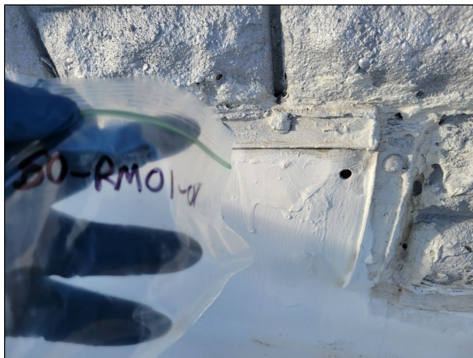
Photo 44. RM01: Roofing material covering the white flat roof
