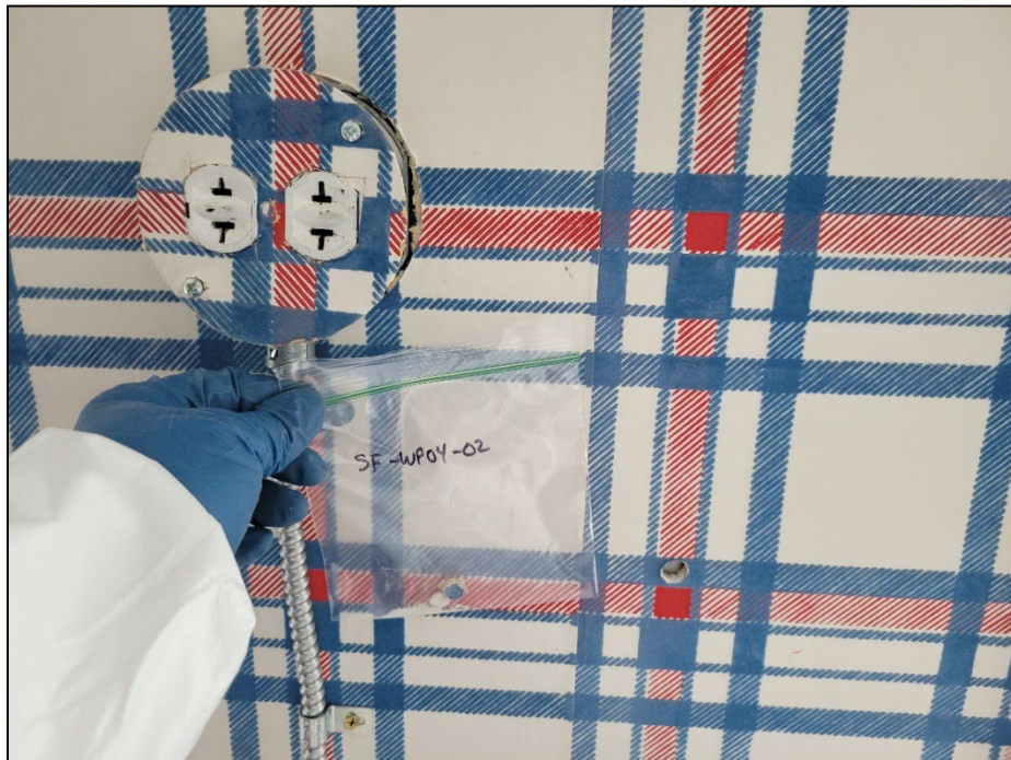
Photo 76. WP04: Red, white, blue wall paper and drywall first floor
