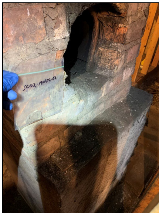
Photo 37. MOR02: Mortar in basement under Montana room
