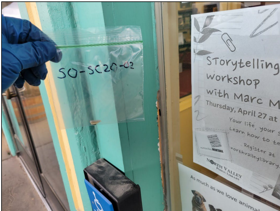
Photo 64. SC20: Silicone outside of main library entrance windows
