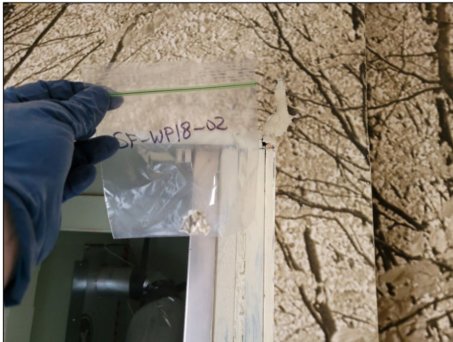
Photo 90. WP18: Trees wall paper and drywall first floor
