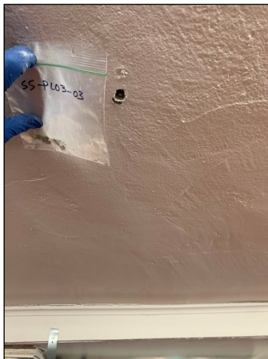
Photo 41. PL03: Plaster ceiling in main library room
