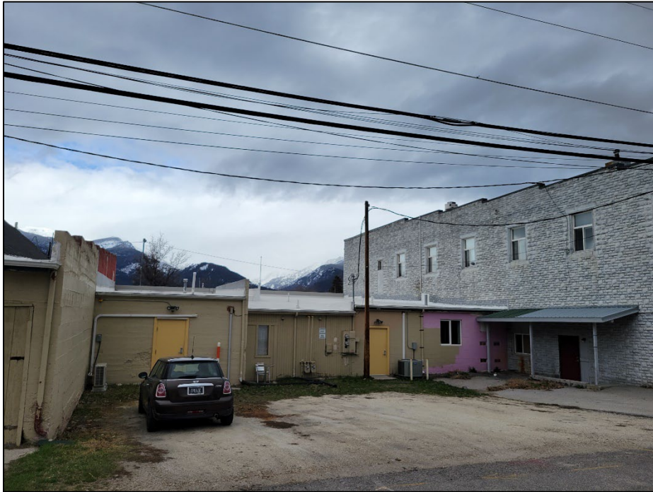
Photo 5. April 11, 2023. Outside looking west: The two yellow doors are employee entrances / emergency exits from the library. Concrete wall between second story and left yellow door. Block walls on majority of tan and pink walls. The ground between the building and alleyway are soil covered and receive the entire run off from the roofs.
