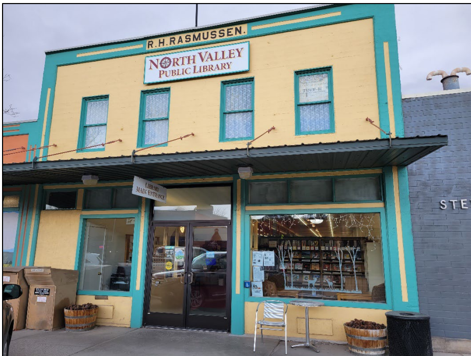
Photo 2. April 11, 2023. Outside looking east: The main entrance to the library.
