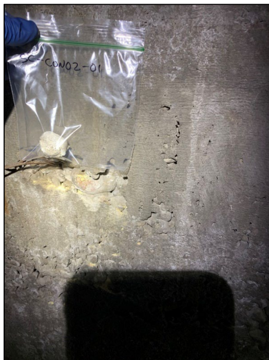
Photo 7. SO-CON02: Concrete in the basement under the front desk
