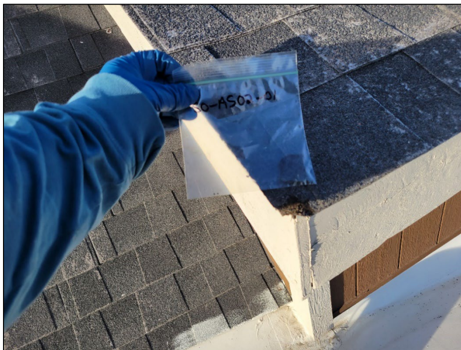
Photo 1. AS02: Asphalt shingles
