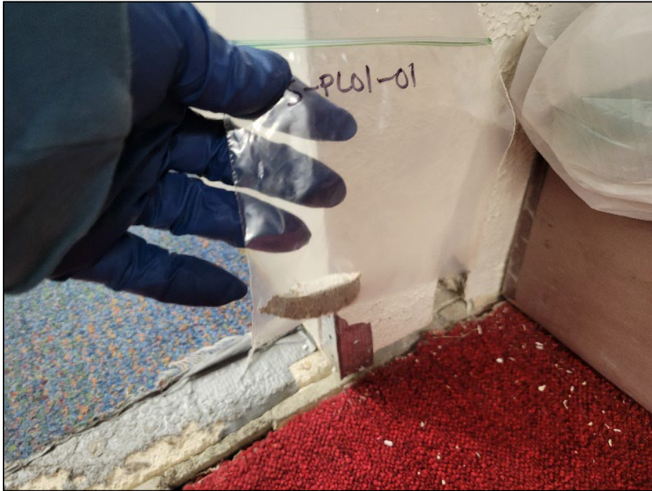
Photo 39. PL01: Plaster wall in main library room
