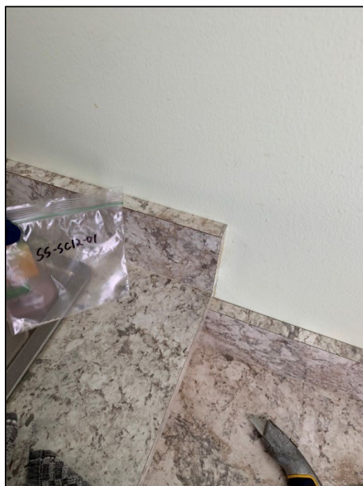
Photo 56. SC12: Silicone in kitchen / staff break room
