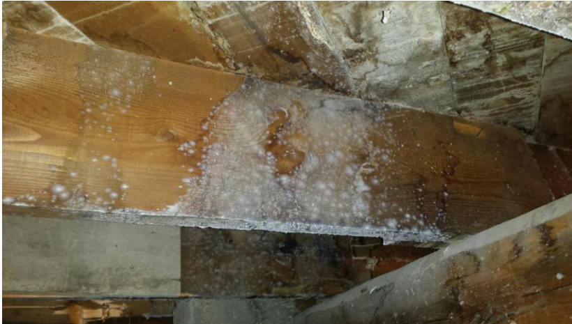
There is a lot of visible mold growth on the floor joists and plank sheathing.
