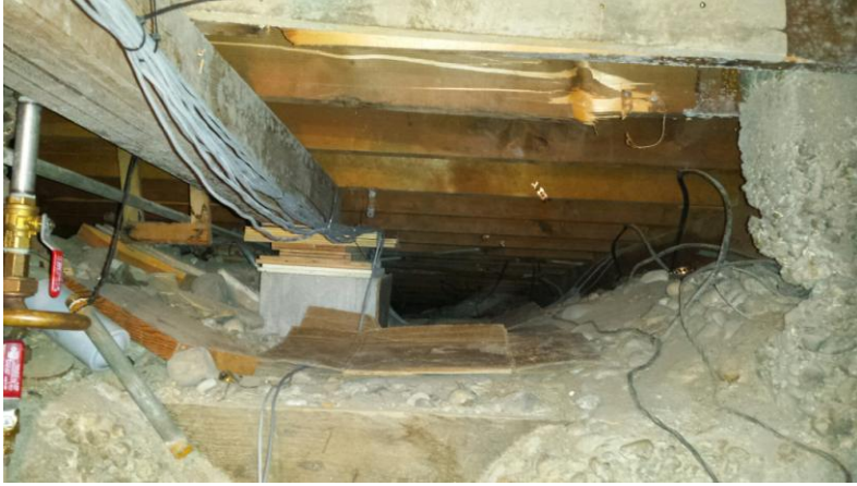
There is a lot of visible mold growth on the floor joists and plank sheathing.
