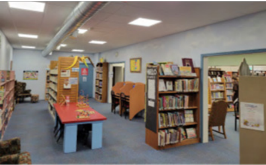
Figure 6: Lack of separation between areas
