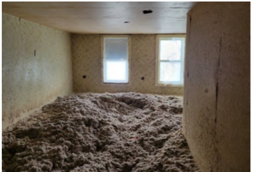
Figure 11: Upstairs Room filled with insulation
